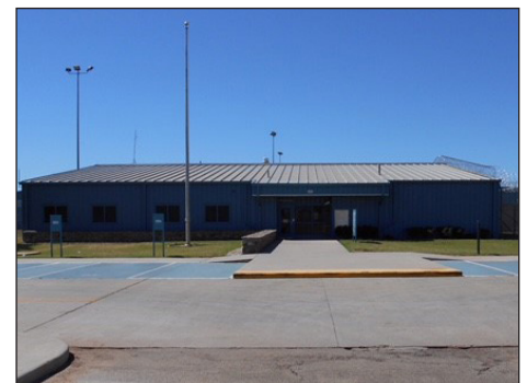
Ware Transfer Facility in Colorado City.
