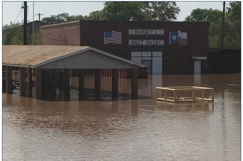
Flooding at the Ramsey Unit.
